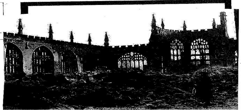
The cathedral demolished.
